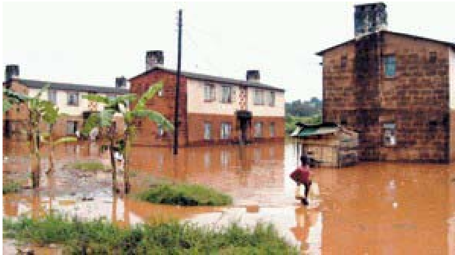
Plate 5.2: A flooded housing Estate constructed in a wetland
