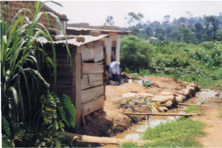
Plate 7.5: Use of Earth Bags against flood waters in a wetland.
