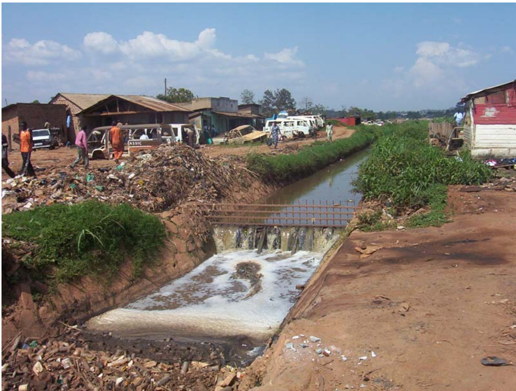
Plate 6.4: A blocked drainage channel due to inappropriate solid waste management practices
